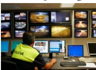
Control center (police building)
